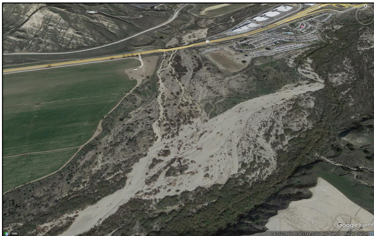
Above: Aerial imagery of widened floodplain along the Utom River hosting riparian scrub and woodlands. (Photo obtained from Google Earth 2022.)
