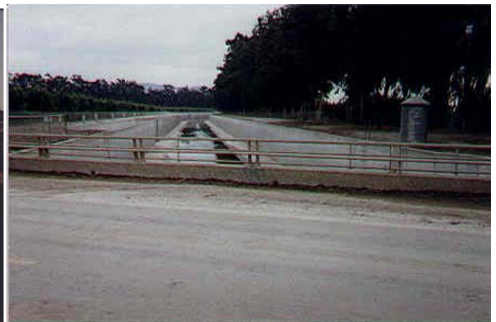
Site 3. Revolon Slough at Hueneme Road bridge, up-gradient.
