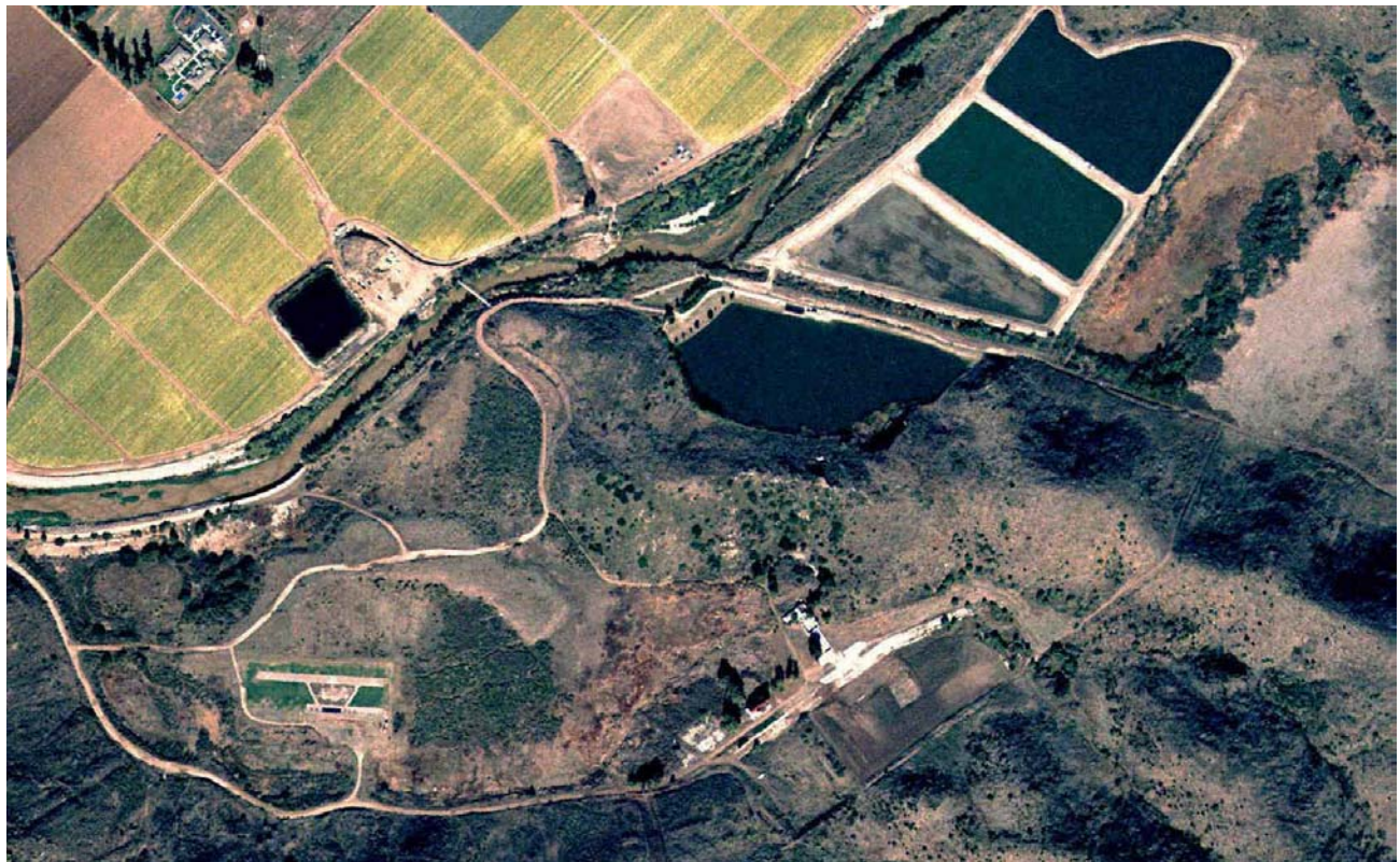
Figure 23. Aerial Photograph of Calleguas Creek at Camarillo Regional Park (Site 34)
