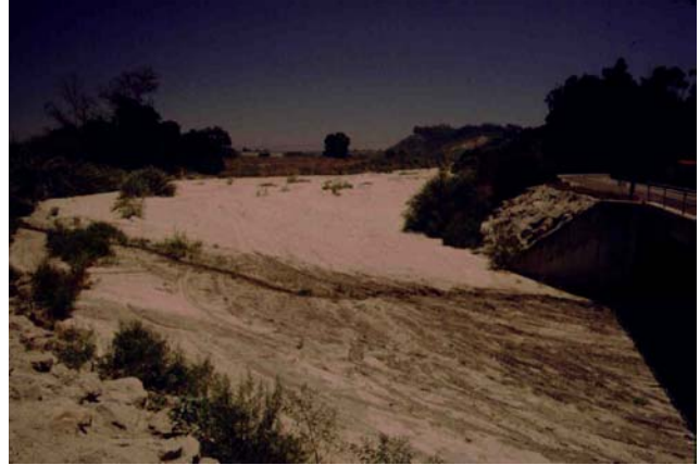
c. View upstream from St. John's Seminary Road of bed full of sediments
