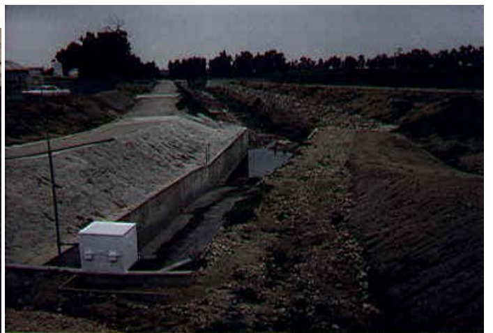
Site 7. Unnamed tributary at La Vista Avenue bridge, down-gradient
