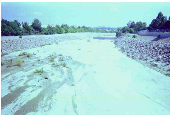
Site 24. Calleguas Creek at Adolfo Road bridge, down-gradient.
