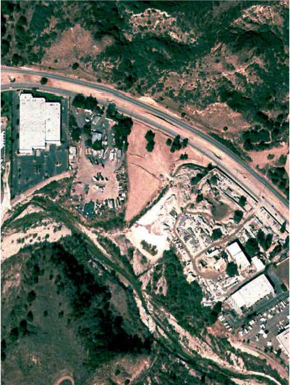
Figure 36. Aerial Photograph of Arroyo Simi at Simi Recycling Center (Site 18)
