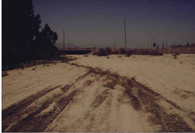
a. View downstream towards Upland Road of channel bed full of sediments and little vegetation.
