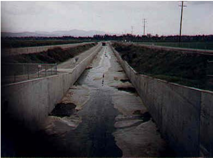
Site 5. Beardsley Wash at Central Avenue bridge, up-gradient.
