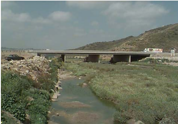
b. View upstream towards U.S. 101 bridge. Channel bed is routinely dredged by Ventura County Flood Control District.
