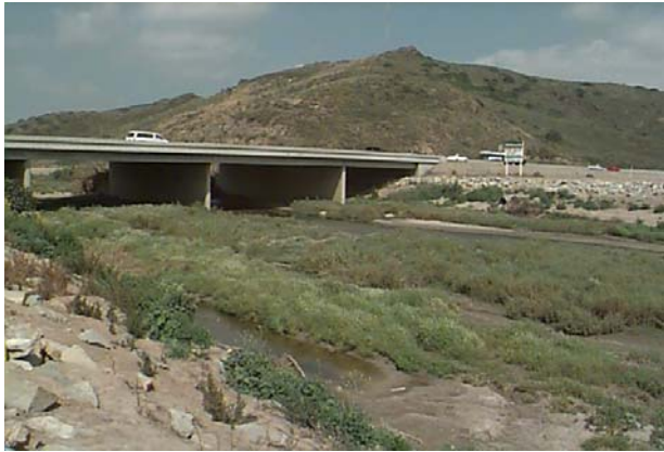
a. View north at U.S. 101 bridge over Arroyo Conejo
