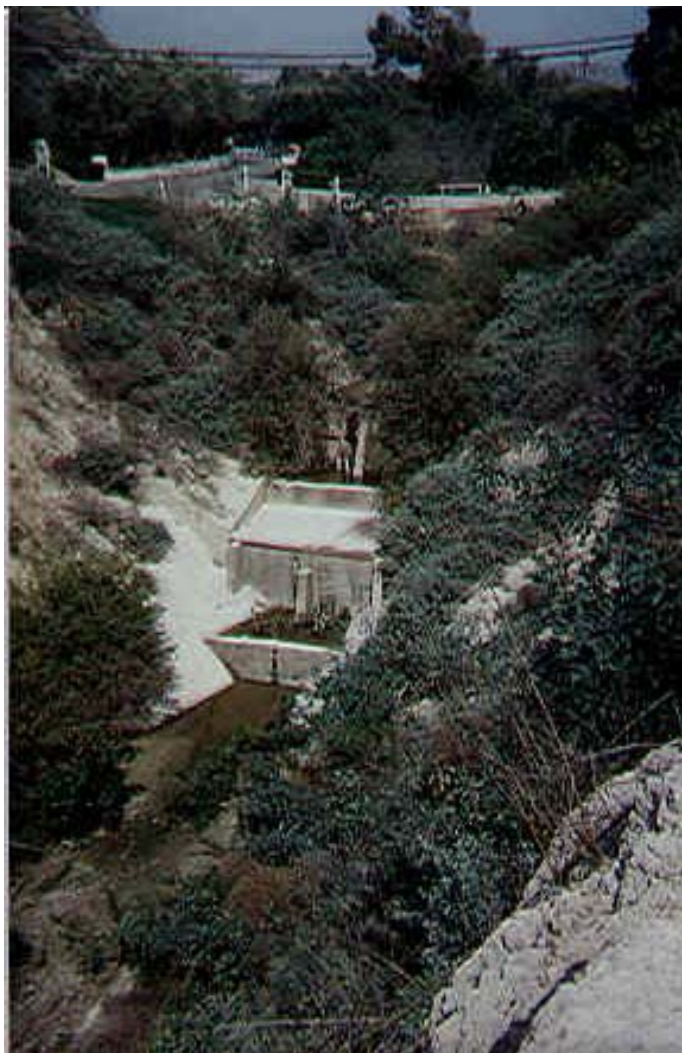
Site 12. Coyote Canyon at Bradley Rd. crossing, down-gradient
