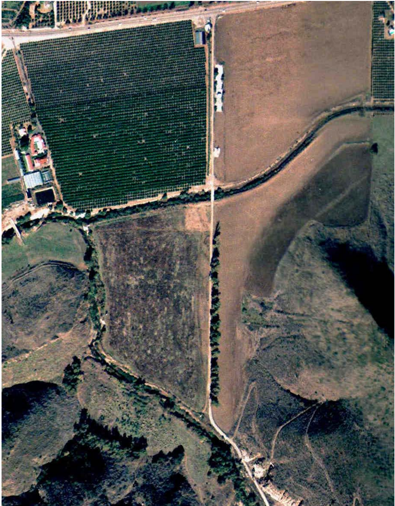
Figure 34. Aerial Photograph of Arroyo Santa Rosa at Arroyo Conejo (Site 30)
