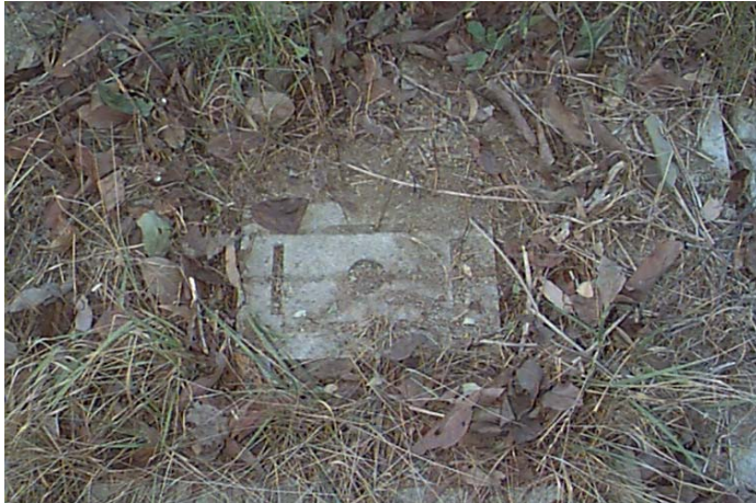
Site 14-Photograph 3. Example of slope stabilization material.
