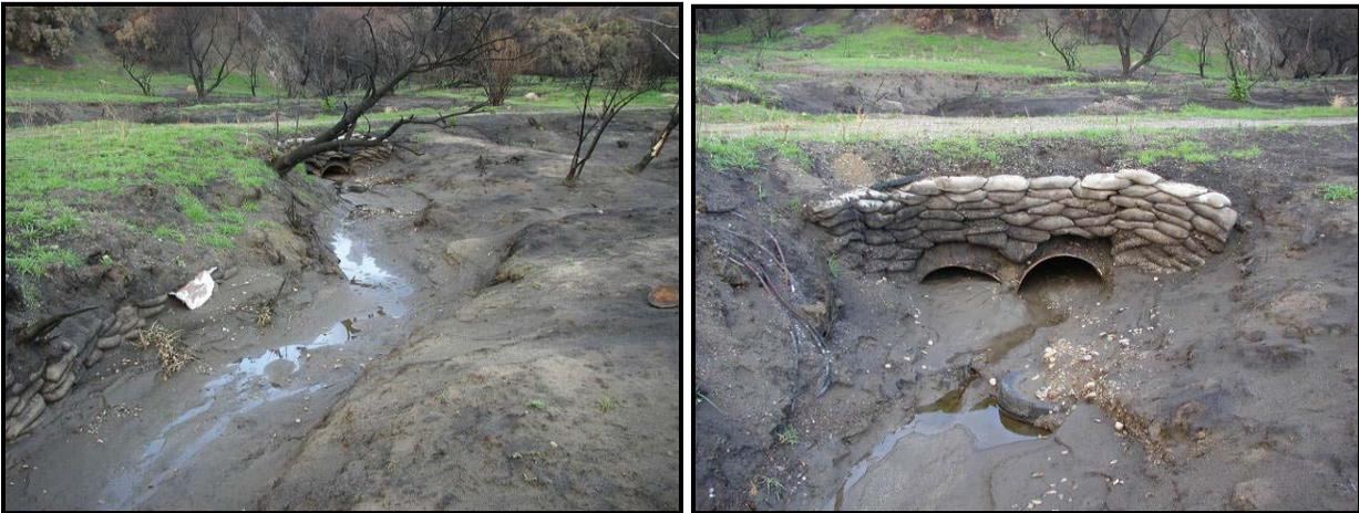
Sandbag bank stabilization and an old culvert crossing on Lyon Canyon Creek (23Feb2004).
